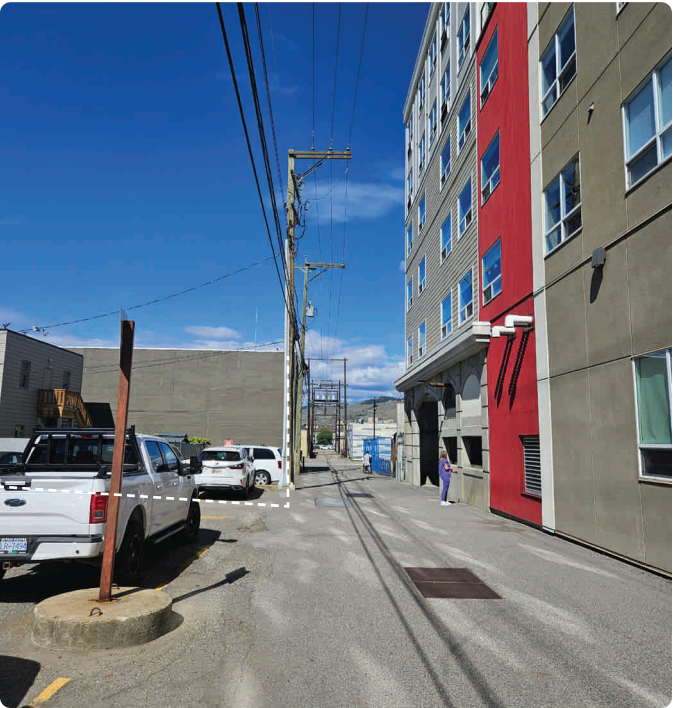
Figure 03 Hydro Line and Transformer at Lane PL
