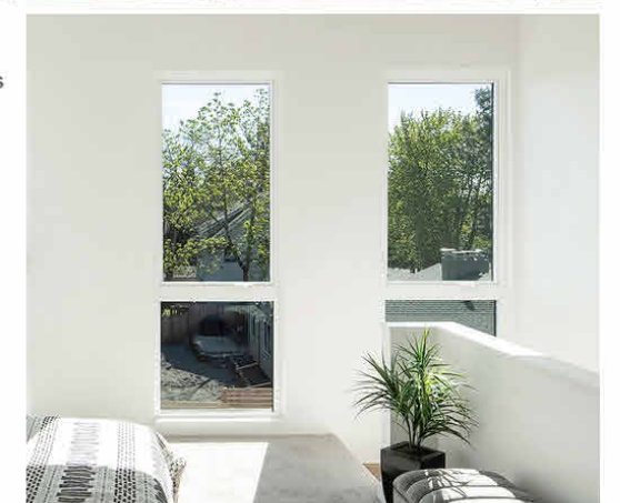
Maximize natural light with large windows. Top hung awning windows meet BC Housing standards and ensure code compliance where a drop exists of more than 1.8m
