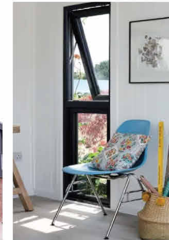
Maximize natural light with large windows. Top hung awning windows meet BC Housing standards and ensure code compliance where a drop exists of more than 1.8m
